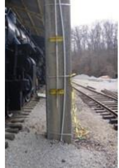
Abbott Bldg. Power Switch
